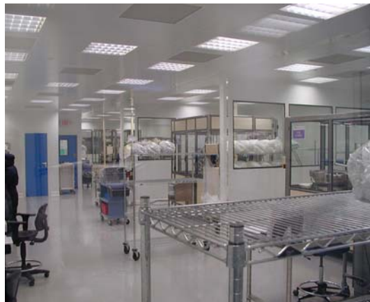
Clean Room Construction
